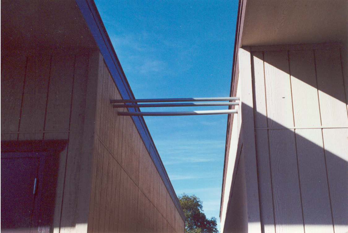
Figure 7: Electrical Conduits running between Portables
