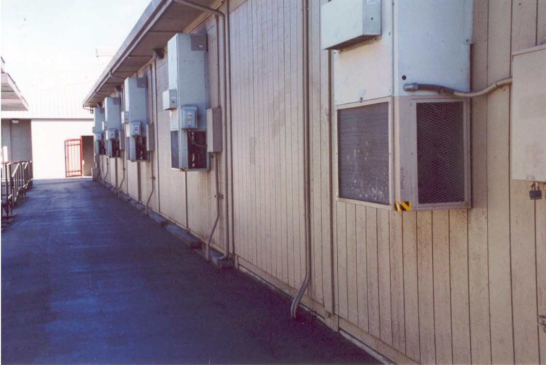
Figure 5: Rear Wall of Classroom numbers 15 to 19
