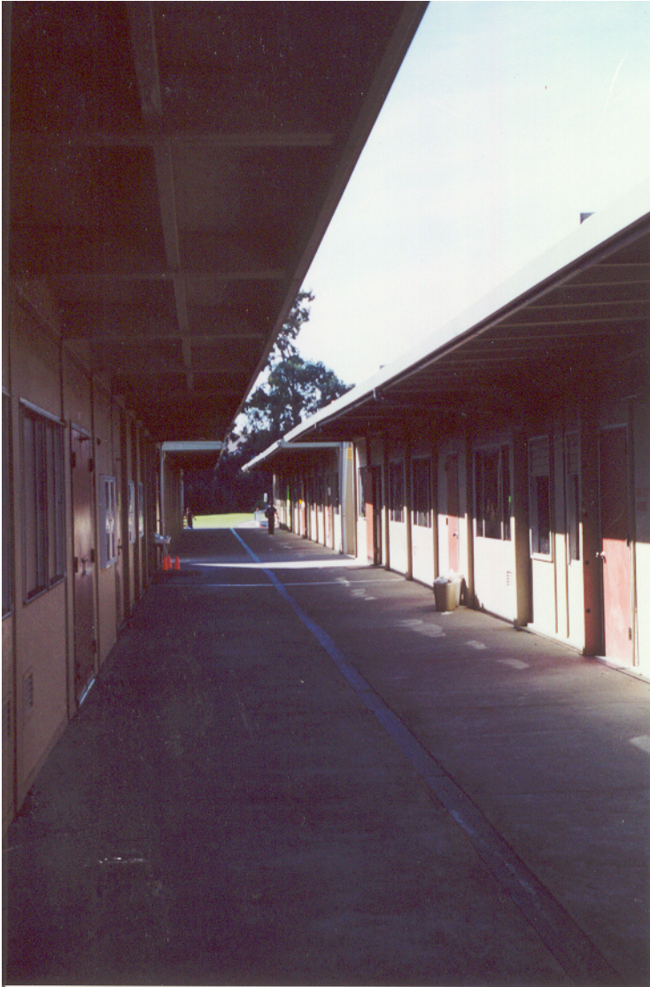
Figure 9: Front Entrance of Classroom numbers 7 to 10 & 11 to 14
